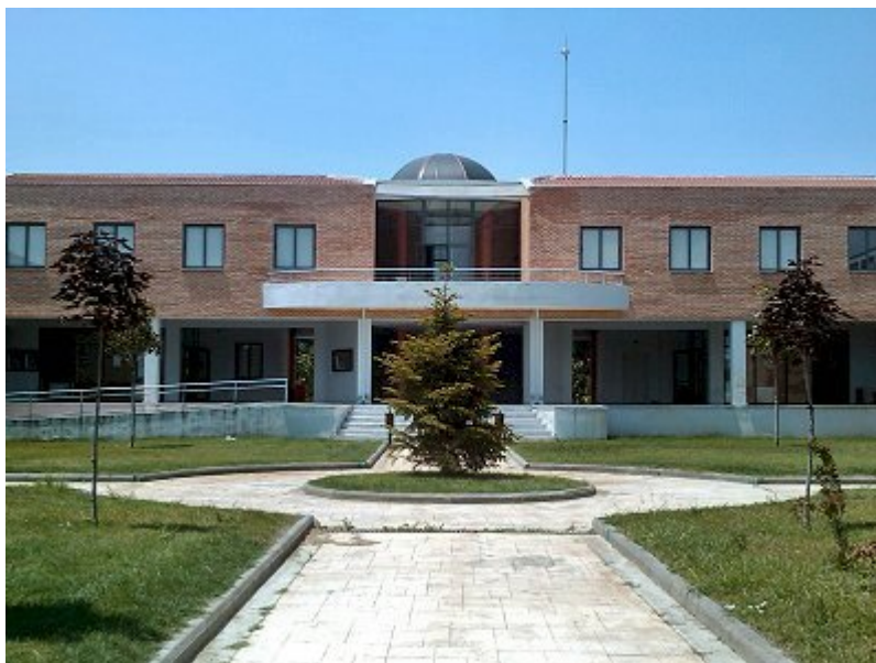
Figure 2. View of the Department's building
